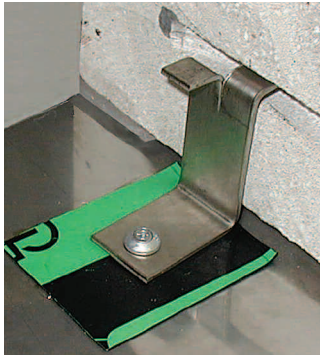
Figure F. Split-tail anchor
